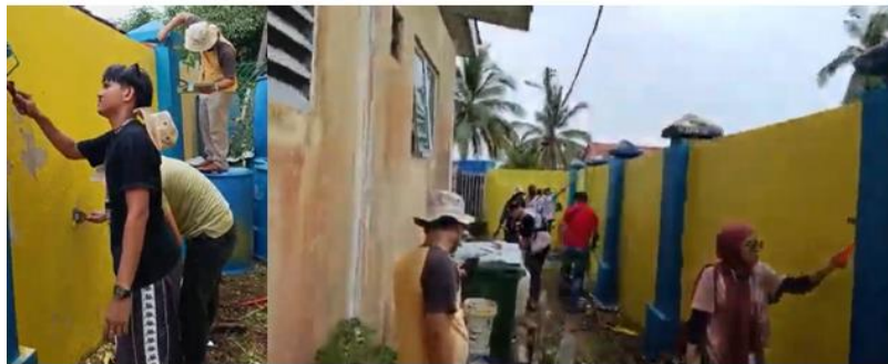
Figure 2. Repainting Activities at the Royal Malaysian Customs Academy, Kampung Tanjung Surat
