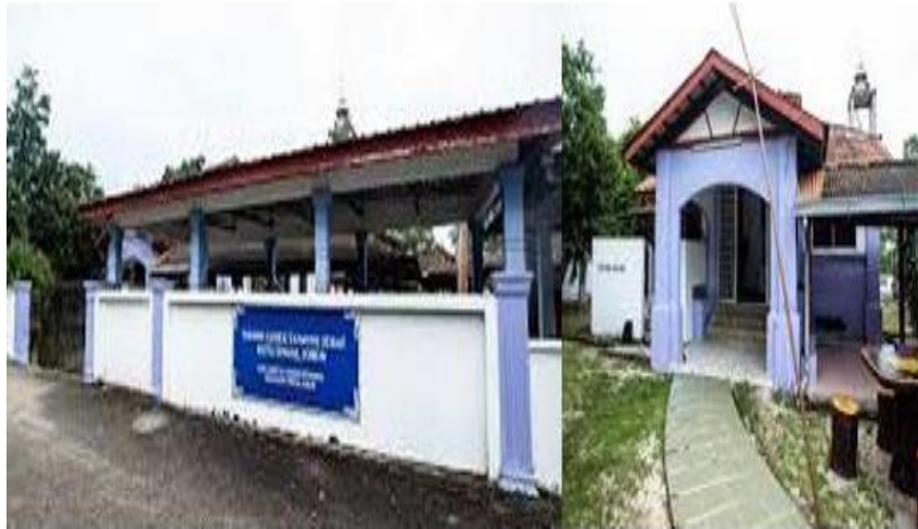
Figure 4. Mosque Yard Clean-Up in Kampung Tanjung Surat, Johor, Malaysia
